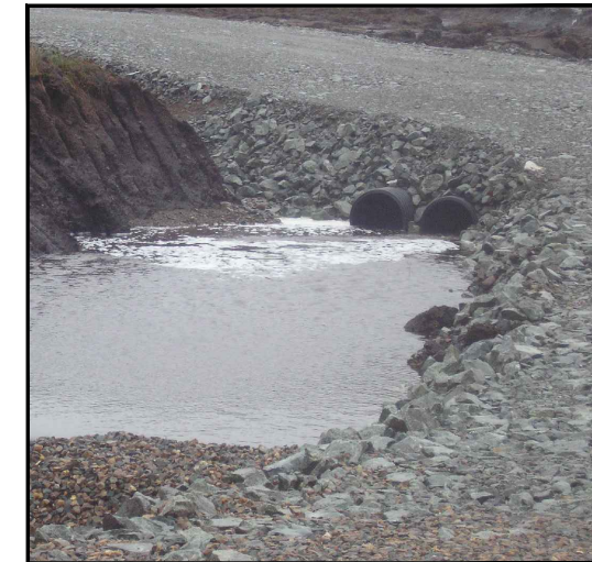
TYPICAL UNDER TRACK DRAINAGE
