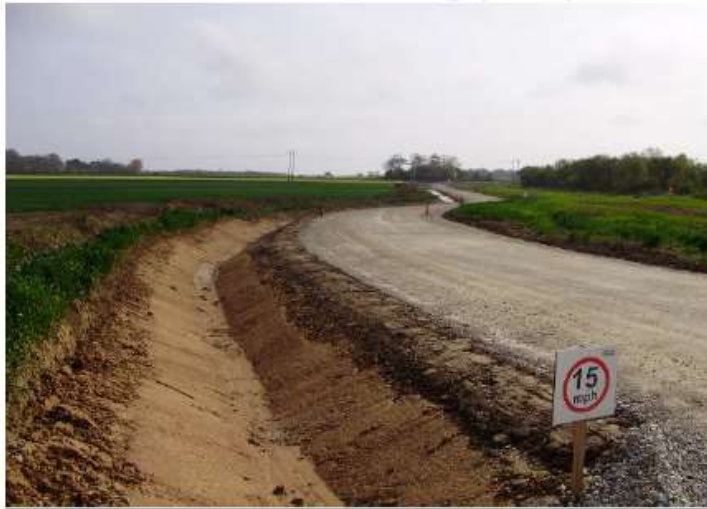
GP - SuDS construction awaiting check dam reinstatement
